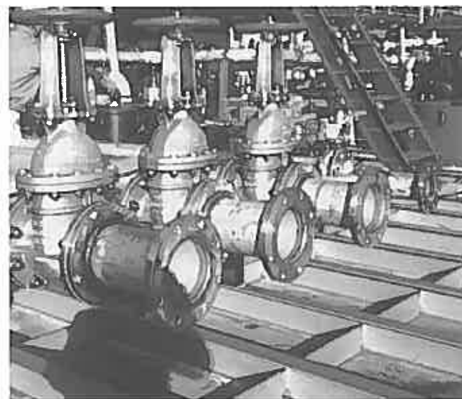
Fig. 2 - An application of DW-316L for fillet welding of the pipefitting of a chemical tanker.
