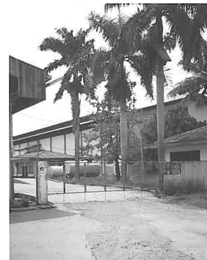
Fig. 2 - The INTIWI's factory in Tangerang started the production of electrodes in 1977 and recorded a production of 19,000 metric tons in 1997. Their persistent quality control earns a high reputation among users. Mr. Sumarno, the successor of Mr. Gunawan, has been engaged in management of the production for more than 22 years.
