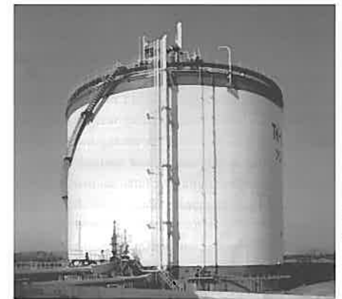
Fig. 4 - Cylindrical LPG storage tank is a typical application of LB-52NS
