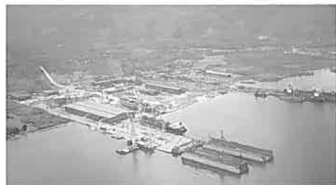
Above: THI Cebu is located on Cebu Island, and is the biggest shipyard in the Philippines
