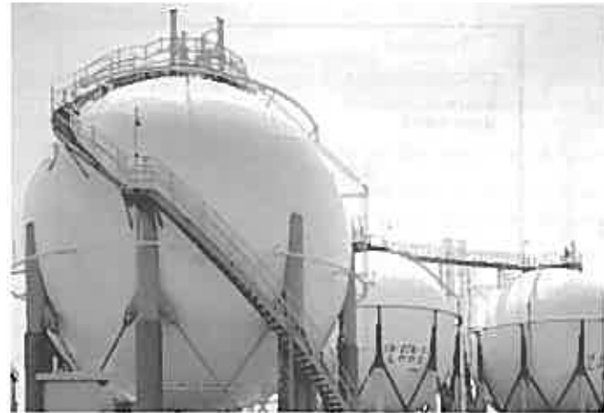
Fig. 1 — Some types of LPG storage tanks use ASTM A537 Cl-2 steel having a minimum tensile strength of 550N/mm 2 , and LB-62L is one of the most suitable covered electrodes for this steel.
