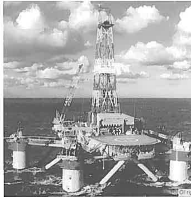
Fig. 1 — Offshore structures require strict notch toughness in order to endure operations in harsh weather and roaring waves.
