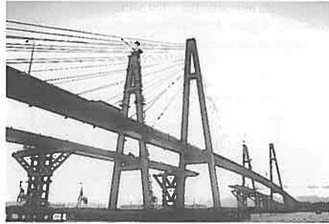
Fig. 1 — Consumption of 590N/mm 2 -class high strength steel is less than that of mild steel and 490N/mm 2 -class high strength steel, but it is an indispensable grade of steel in bridge construction, hence MG-60 is, too.
