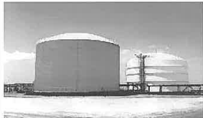
Figure 1. A flat-bottomed cylindrical single shell tank for storing liquefied butane gas is one recent application for NB-1SJ, when constructed per BS7777 specification requiring -50°C notch toughness based on fracture mechanics (Photo courtesy of Toyo Kanetsu K.K.)
