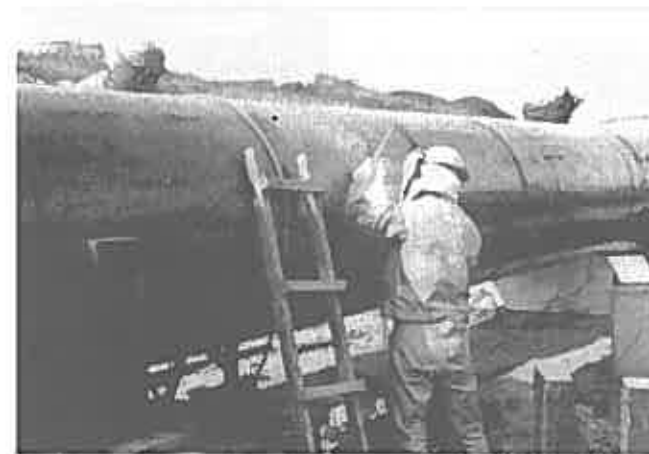
Photo 1. An application of the DL procedure using a vertical-down, low-hydrogen electrode
