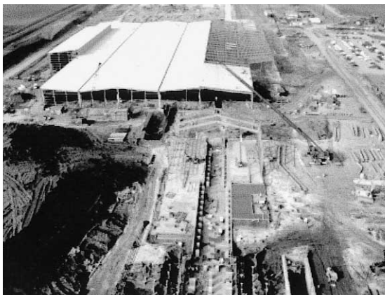
Steel structure PEB in UK
